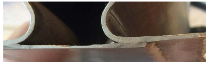
A welded band sealed off the leaking toroid convolution. Brilliant.
