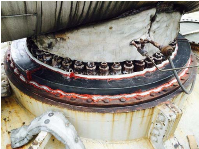
Rolled angle with rope and caulking to seal the gap
