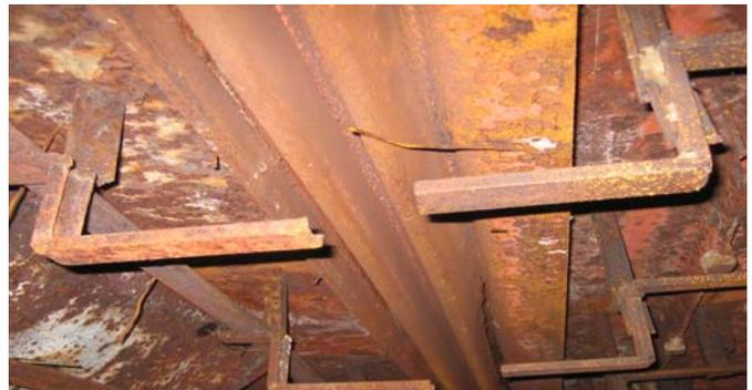
Combustion Engineering (CE) COR-TEN expansion joint - installed 1976
